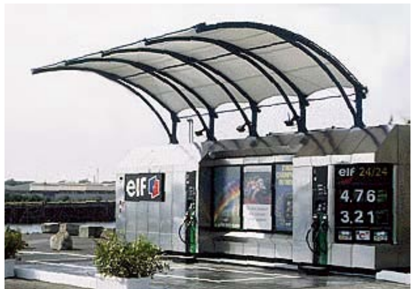
This mobile filling station in Nantes, France has Stage I vapour recovery.
