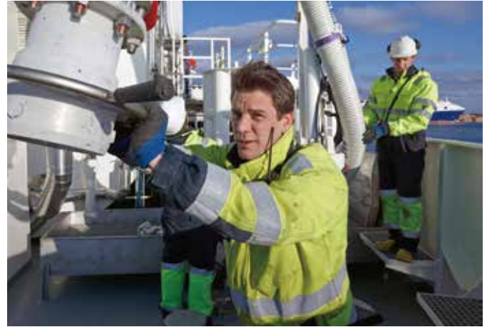
Connection and disconnection of the fuelling hose within one minute was achieved
