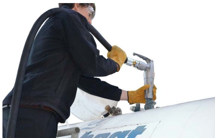
Picture 1: Filling a stationary tank with GG10
